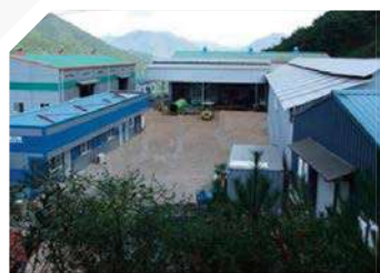
TSA Coating Factory
